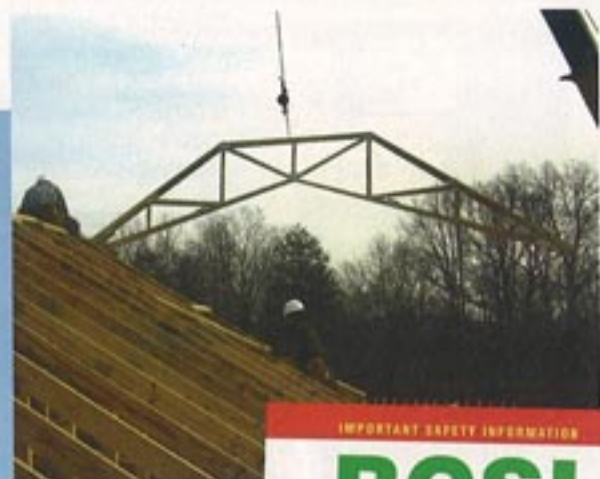
Figure 3. Produced by a consortium of truss manufacturers, the BCSI (Building Component Safety Information) guide is a good source of information on how to safely assemble these unwieldy building components.
